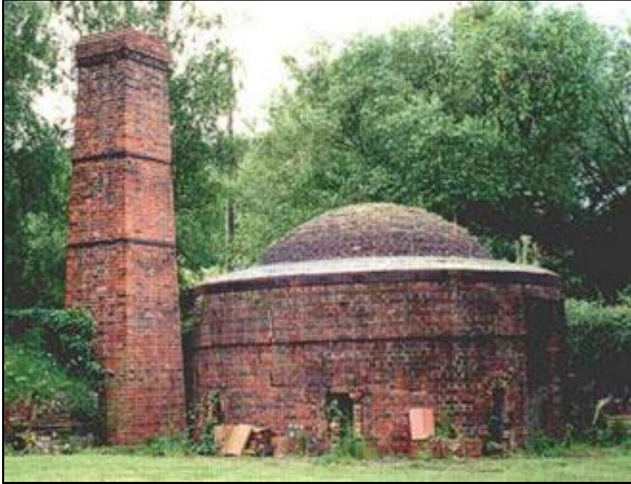
Intermittent burning down-draft type kiln
