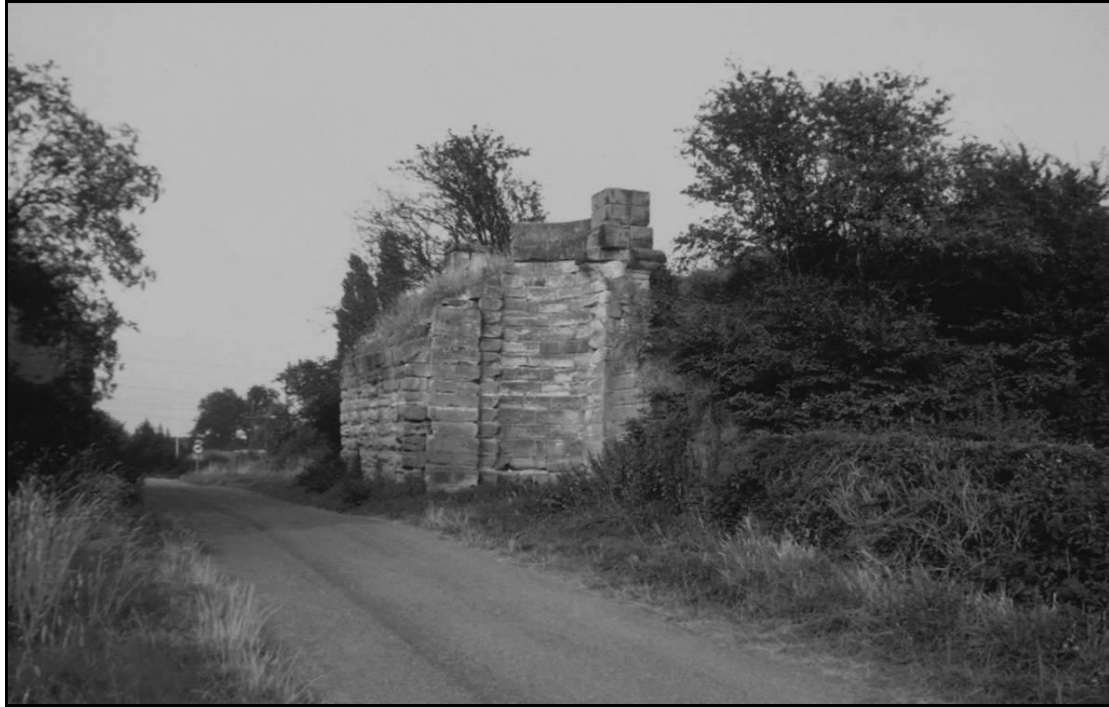
The remains of the bridge built by Joseph Nowell & Sons which carried the Coleorton railway over Aqueduct Lane, Gelsmoor (known colloquially as Akadoc lane)
