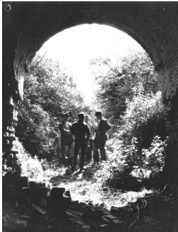
The entrance to the Pegg's Green tunnel at St. George's Hill, Swannington which was built by Joseph Nowell & Sons
