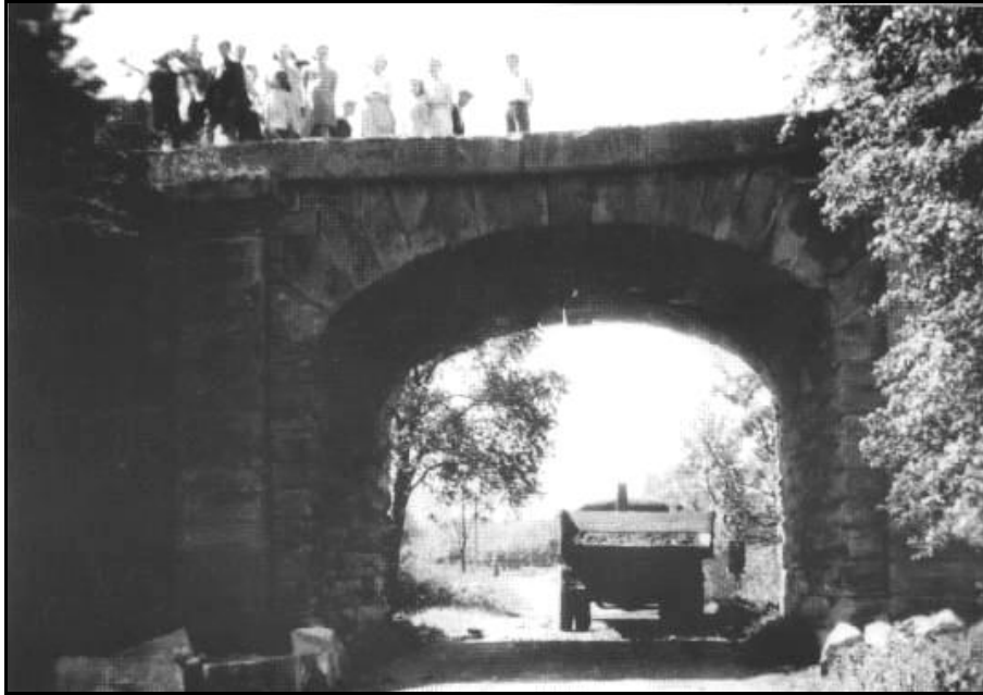
The bridge being demolished
