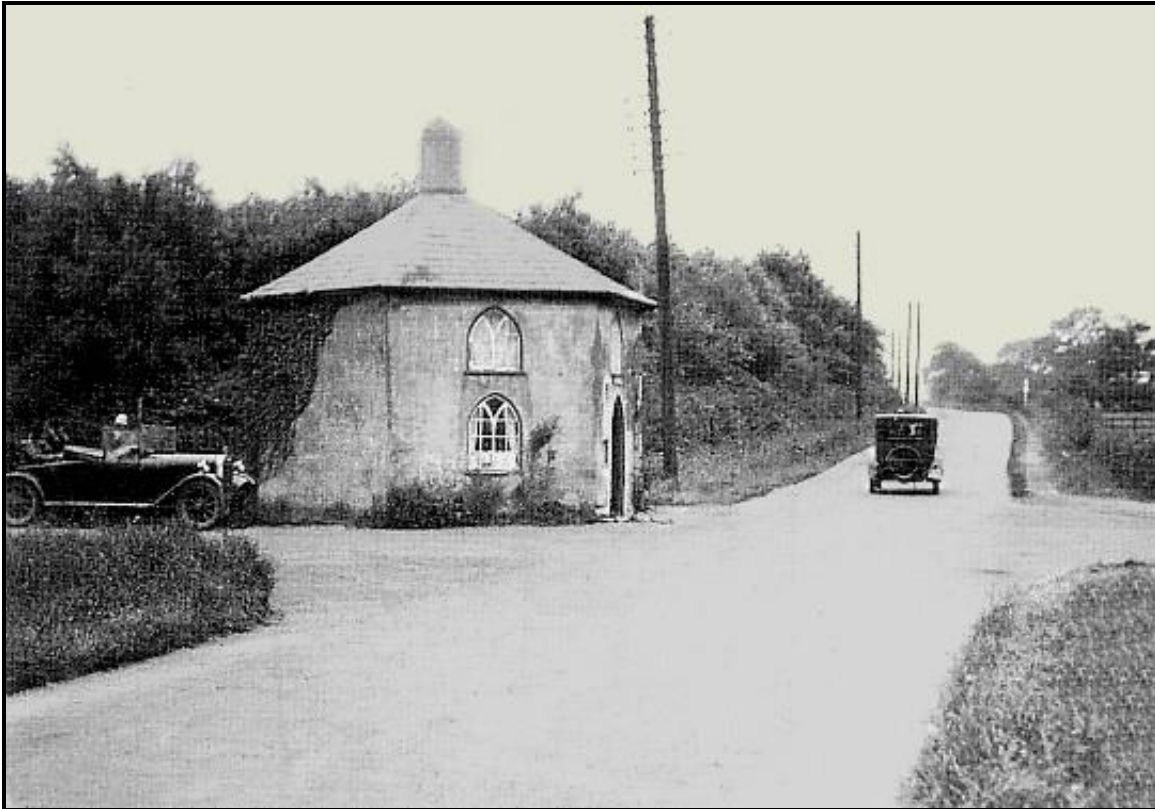
Lount hexagonal toll house pre 1930
