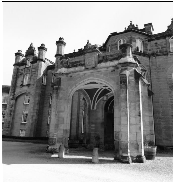
Porte Cochere (carriage porch) with vaulted ceiling
