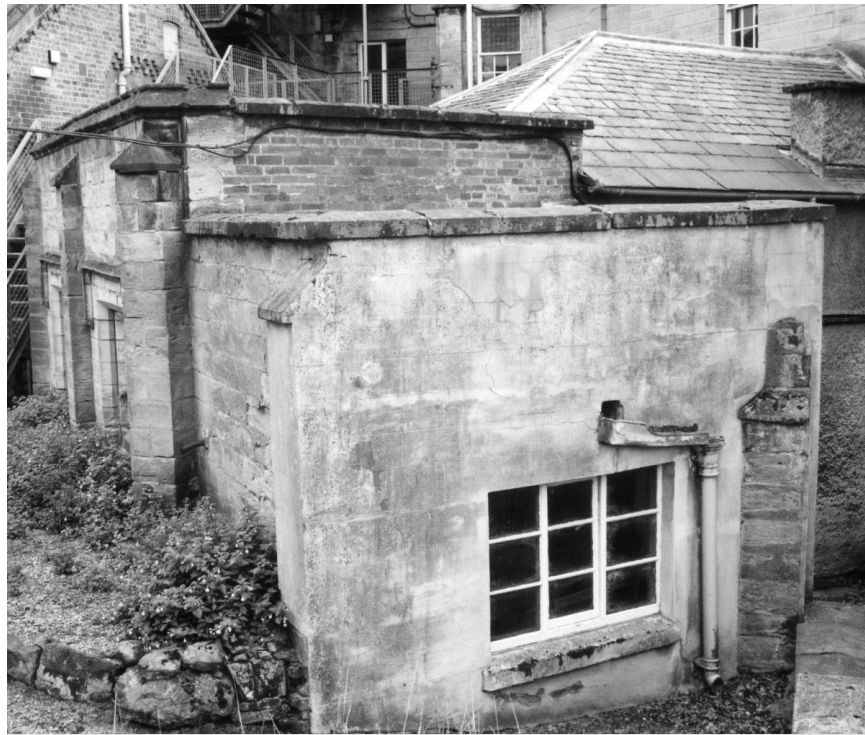
1997 view of churn room and scullery end of dairyhouse
