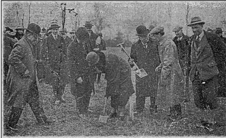
Lady Beaumont turning the first sod on land at Newbold for the “New Lount Colliery”.
