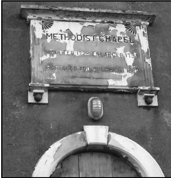
Plaque above front door 2011 METHODIST CHAPEL ERECTED 1778 ENLARGED 1791 RESTORED AND ENLARGED 1862
