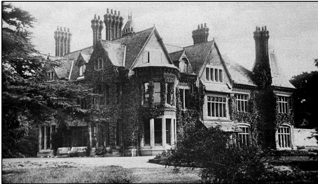
Broom Leys VAD Hospital building
