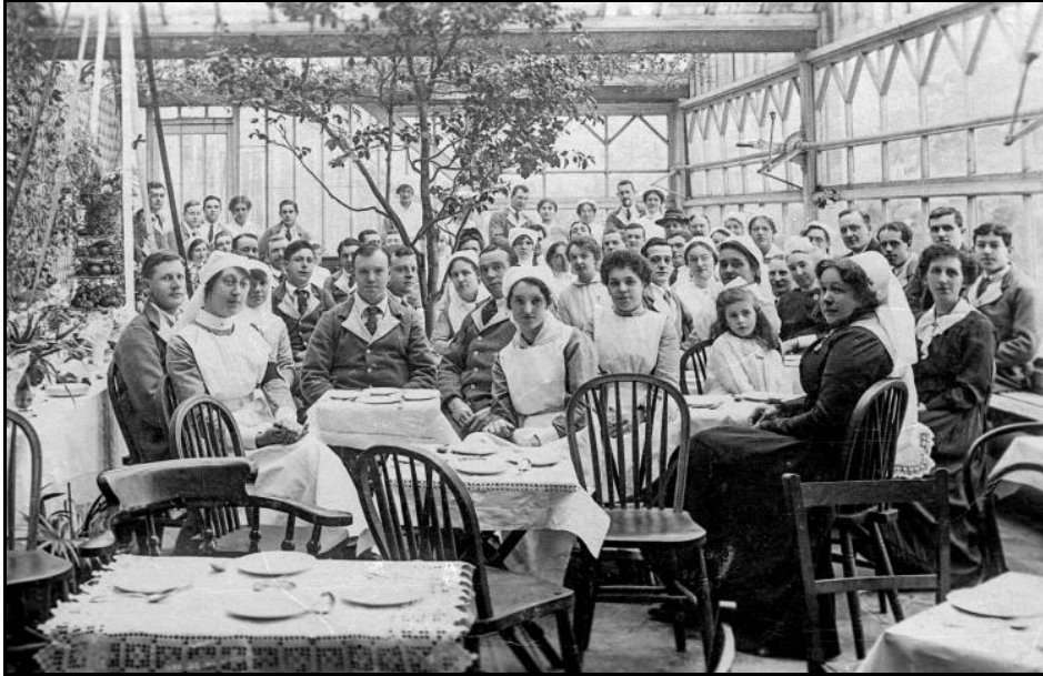
Interior of Broom Leys VAD hospital
