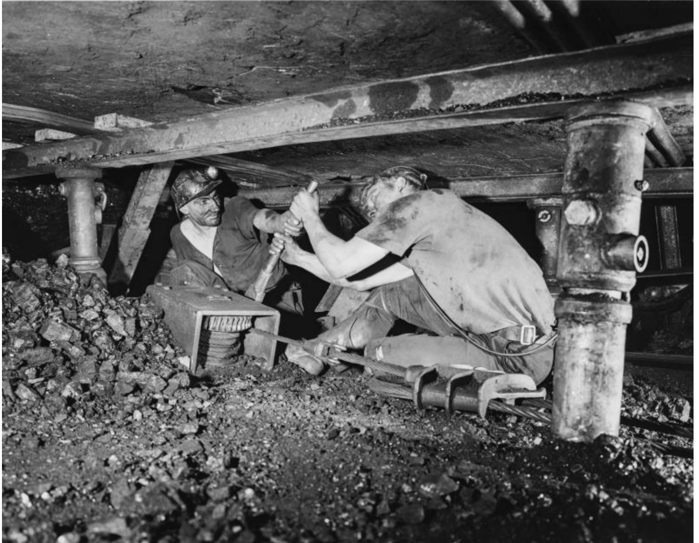
Underground at New lount Colliery
