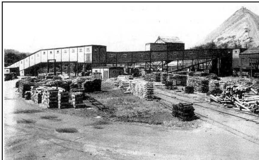
The above photograph taken c.1957 shows the structure which housed the conveyor belt taking the coal from all the seams to the screens which had opened a couple of years earlier
